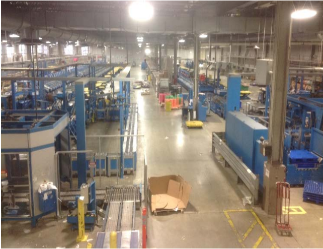
Chicago Tribune's Freedom Center North 115,000 square foot production facility was filled with production equipment that had to be quickly removed & stored.
